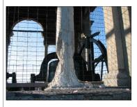
The 8 structural columns have to be replaced along with the balusters and rails.
